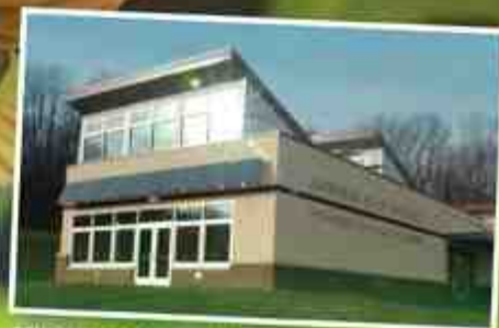
FSU's off-grid Sustainable Energy Research Facility
